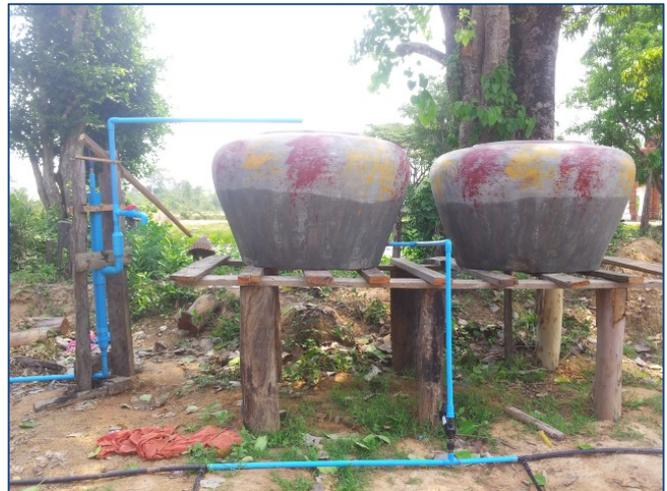
*Connection of water-pipe system, pcv pipe, pump and water jars*
